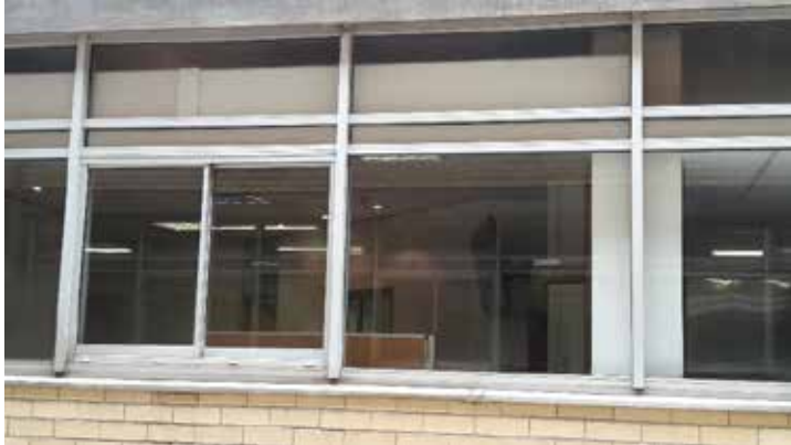
Figure 8: Windows closed, sliding windows and fan-lights
