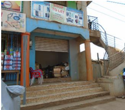
Figure 6: Inaccessible phone/computer repairs shop
