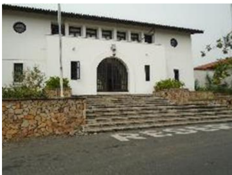
Figure 5: Inaccessible entrance to a building
