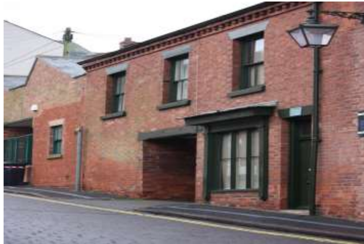
Fig. 1. 8A Victoria Street, Eastwood, Nottingham (Source: author's own photograph)
